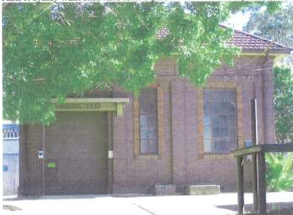
Photo 3: Sydney Water brick valve house adjoins the southern boundary of the site.
